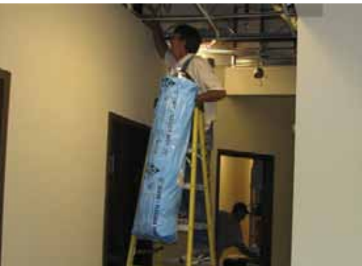
Construction continues in the Municipal Center.
