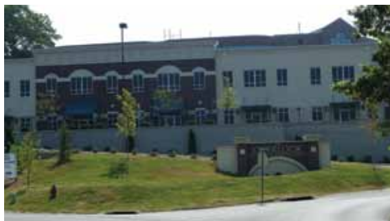
Overlook Park Office Building, located at 212 Overlook Circle, is a new two-story, 22,464 sq ft general and medical office building.
