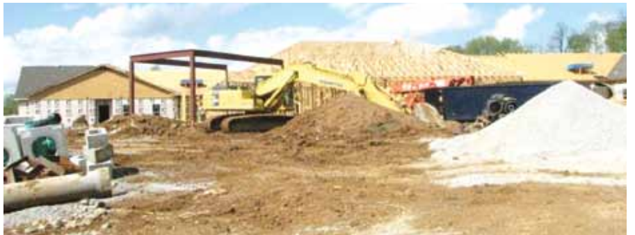
Morning Pointe of Brentwood Assisted Living facility under construction
